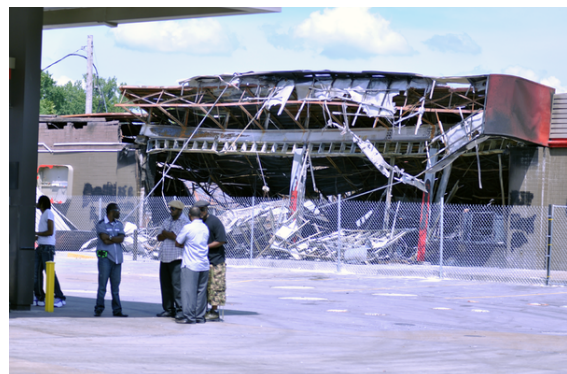
The looted, burned-out QuikTrip gas station in Ferguson.
